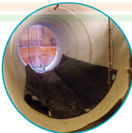
Placing – pillow plug should be positioned horizontally
