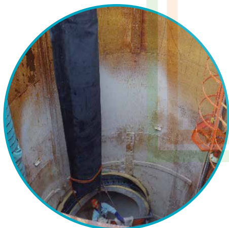
Inserting a folded pillow plug
